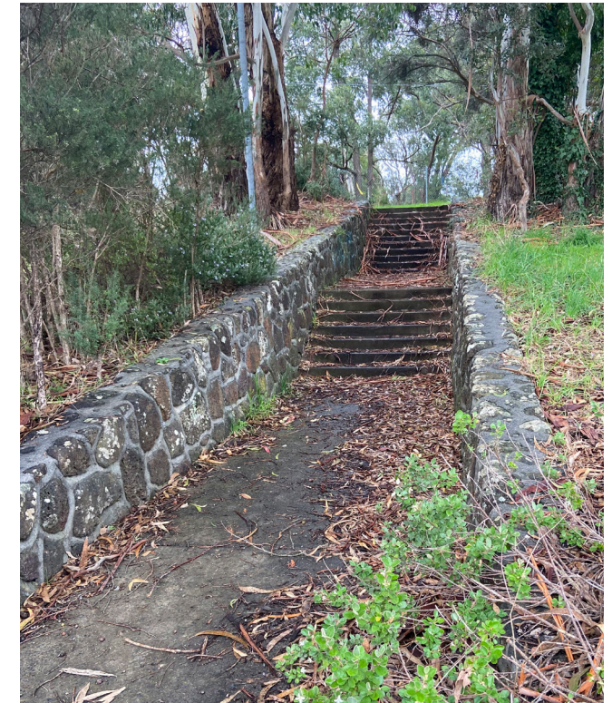
Photo 8 Remnant bluestone staircase
