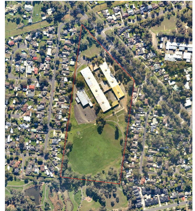
Figure 4: Aerial photo 2014 – showing school buildings
