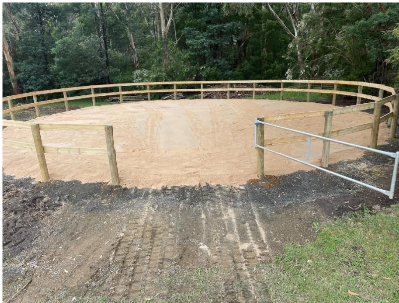
Upper Yarra Pony Club - Leveling, fencing and surfacing of round yard
